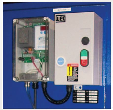
Magnetic starter with auto pulse controls
