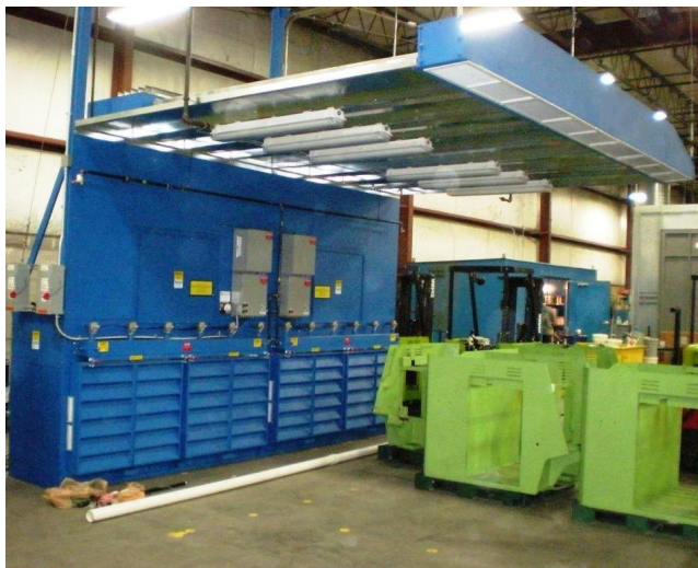
Regain air plenum with no side walls
